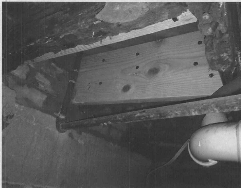
Photo 2 – Joists near fireplace replaced
