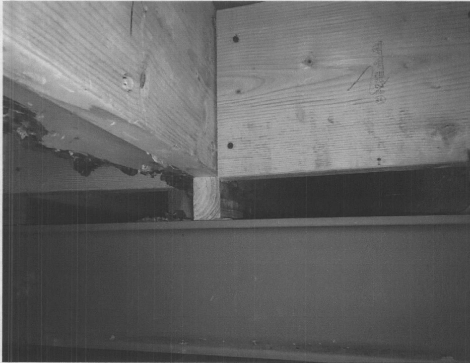
Photo 1 – Bearing block installed tight and bridging replaced
