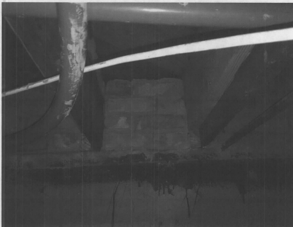
Photo 4 – Typical brick infill
