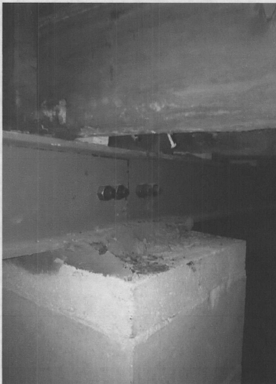
Photo 6 – Interior steel beam bearing condition
