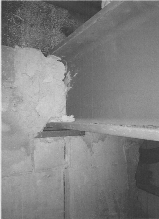
Photo 5 – Steel beam bearing condition at north concrete wall
